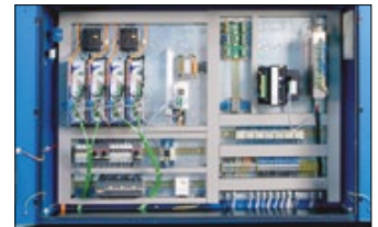
Open and easily surveyed panel includes digital control, cooling fan, transformers and control.
